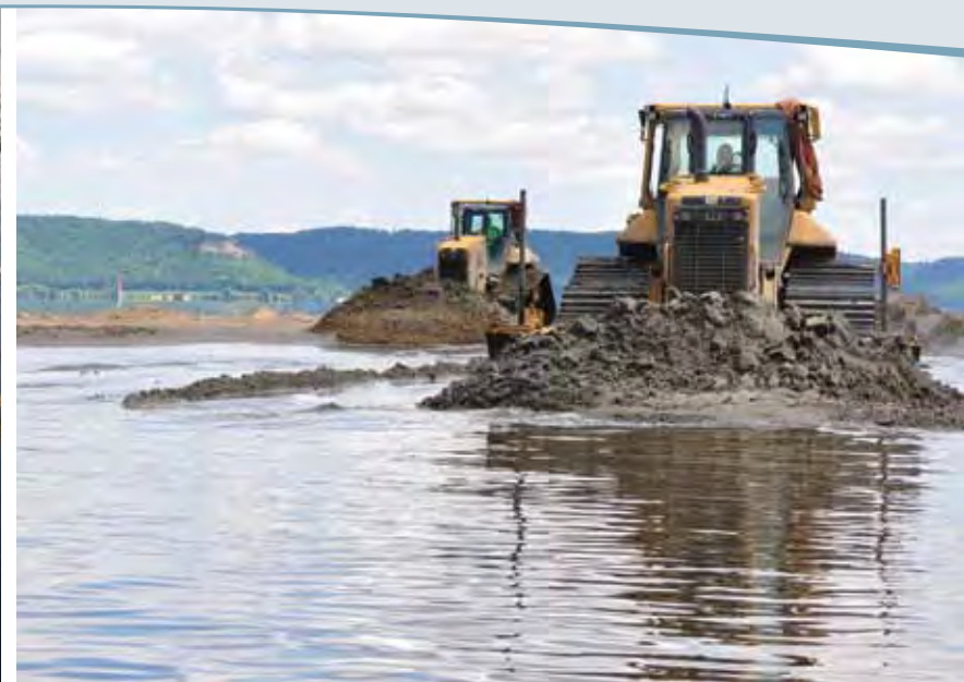
Islands under construction in Mississippi River Navigation Pool 8. RIGHT: A bulldozer helps create a new island as part of a Capoli Slough Habitat Rehabilitation Project.
