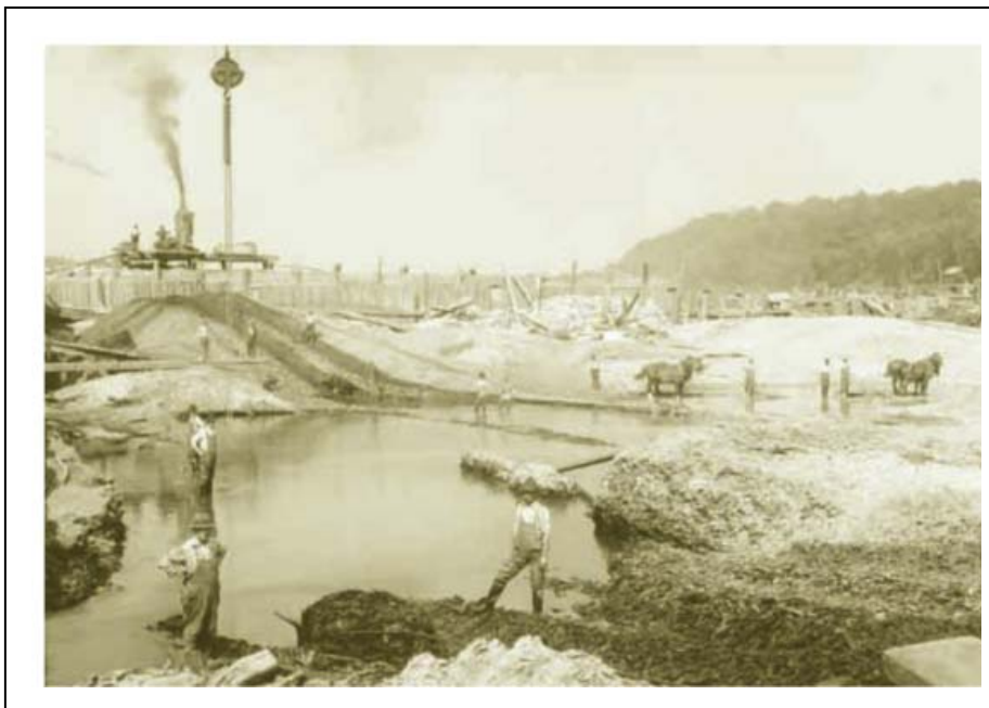
Figure 14. Construction of Lock and Dam 1, 1914 (Source: Minnesota Historical Society)
