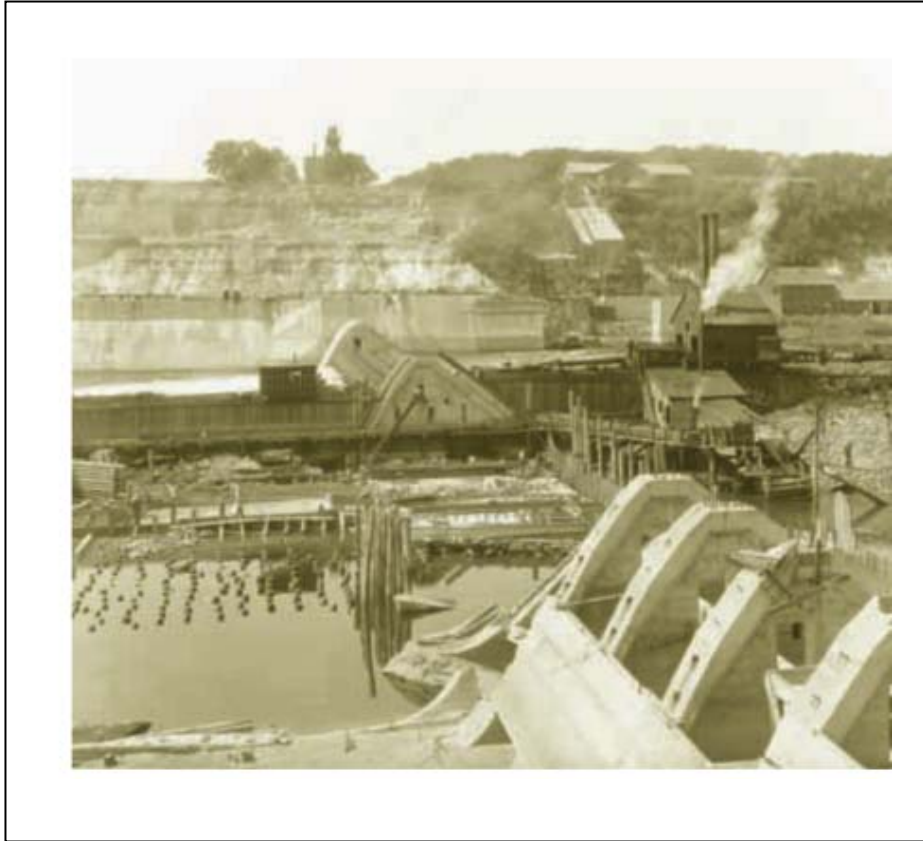
Figure 15. Construction of Lock and Dam 1, 1914 (Source: Minnesota Historical Society)
