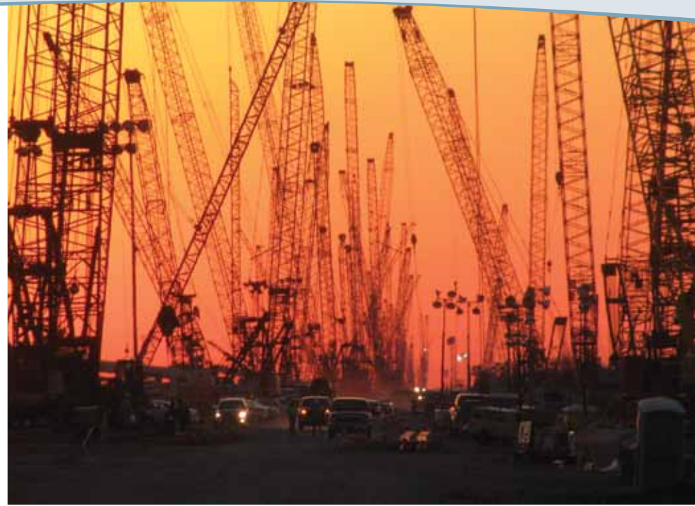
More than 100 cranes fill the skyline of the St. Bernard parish in New Orleans as crews rush to complete construction of 14-foot concrete walls atop existing levees to protect against potential hurricane force waves.
