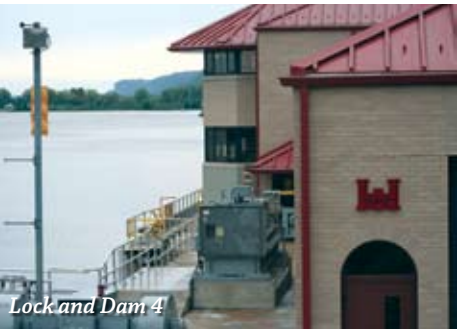
Lock and Dam 4
