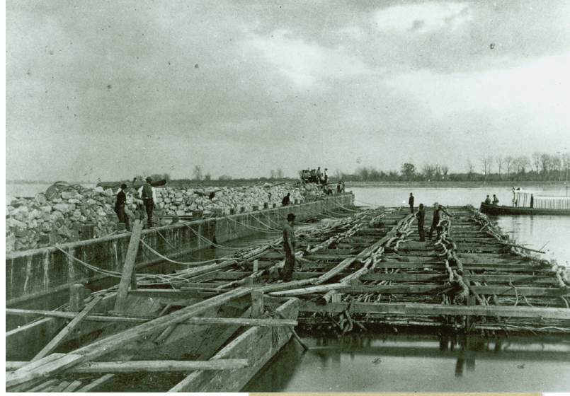
ABOVE, FROM LEFT: Early levee construction, around 1910. Workers construct a willow mat that will be loaded with rock for channel protection or wing dike formation.
