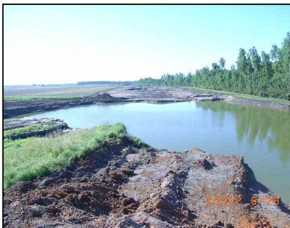
Photograph IV-3. Upper Inflow Crevasses Prior to Repairs
