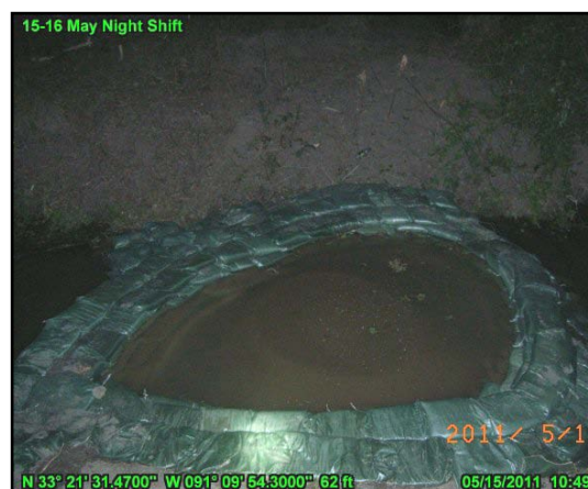
Photograph IV-8. Bagged Sand Boil in Ditch
