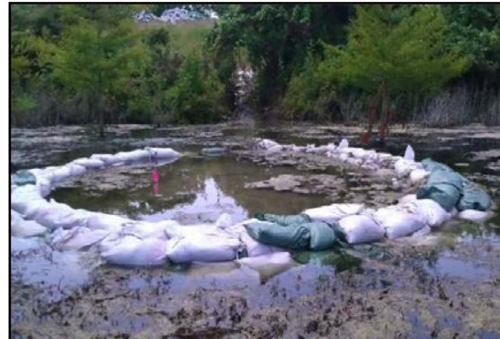
Photograph IV-10. Sandbagged Boils Flowing
