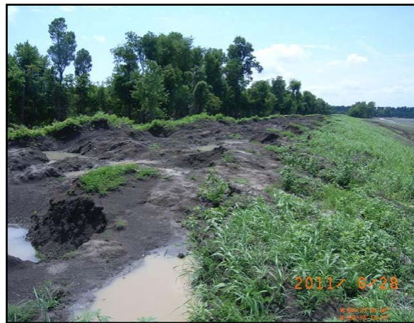
Photograph IV-4. Levee Crown Damaged Due to Overtopping
