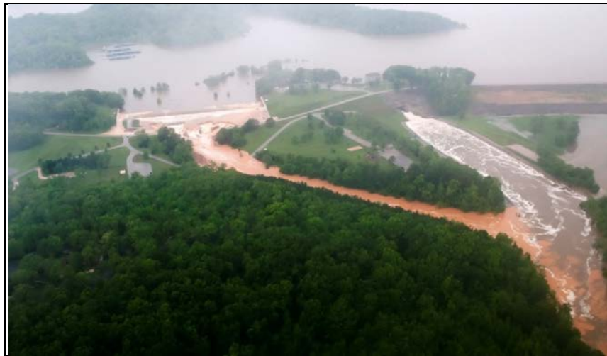
Photograph IV-2. Post 2011 Overtopping of Spillway
