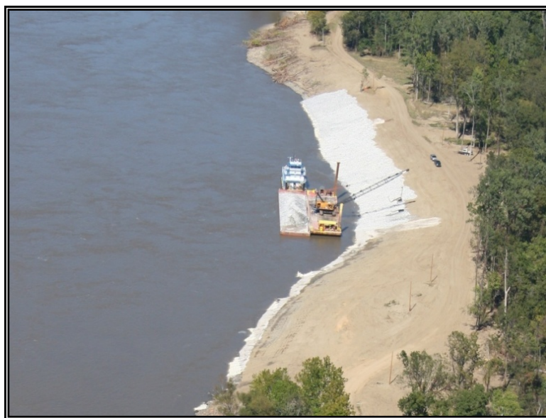
Photograph IV-17. ACM Revetment Under Construction
