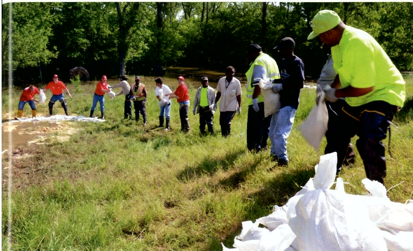
Memphis District (Tenn.) team members form a sandbag relay line with city of Memphis employees during the flood of 2011 to ring a sand boil at the Ensley berm near the USACE Ensley Engineer Yard just south of Memphis. Sand boils occur when water under pressure wells up through a bed of sand, making it look like it is boiling.
