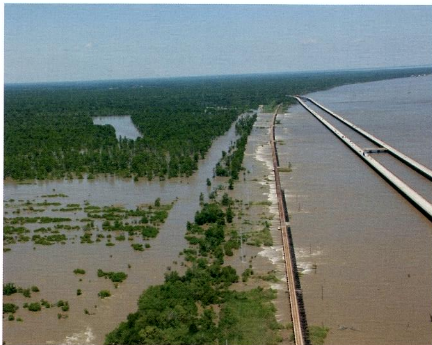
Bonnet Carré Spillway, located about 12 miles west of New Orleans, La., is shown in operation during the 2011 Mississippi River flood. The spillway allows water from the river to flow into Lake Pontchartrain and on to the Gulf of Mexico.
