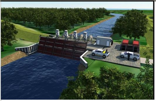
Pump Station Capacity: 1000 cfs (450,000 gal/min)
