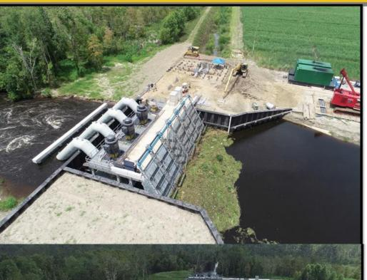
Pump Station Capacity: 1000 cfs (450,000 gal/min)
