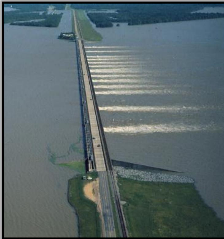
designed under the assumption that the gates would rise prior to river stages reaching 56 feet, all tables, graphs, and data in the water control manual ended at that stage. Thus, rating curves and various equations used by the New Orleans District's hydraulic engineers to extrapolate stages were not as precise as needed, posing an incredible challenge for the district.
