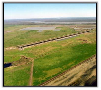
stones. Engineers addressed these problems by placing concrete pads in the outflow channel to reduce future scouring.
