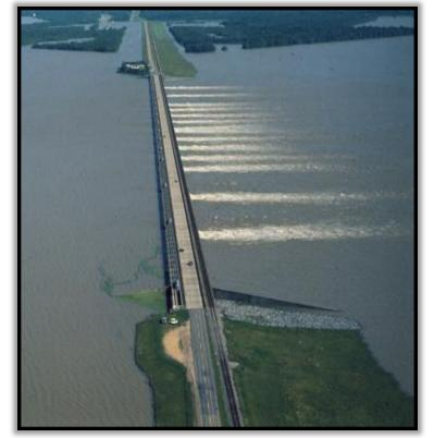
recognized the strong possibility that the river could overtop the gates at the Morganza spillway before reaching the 1.5 million cfs discharge trigger.
