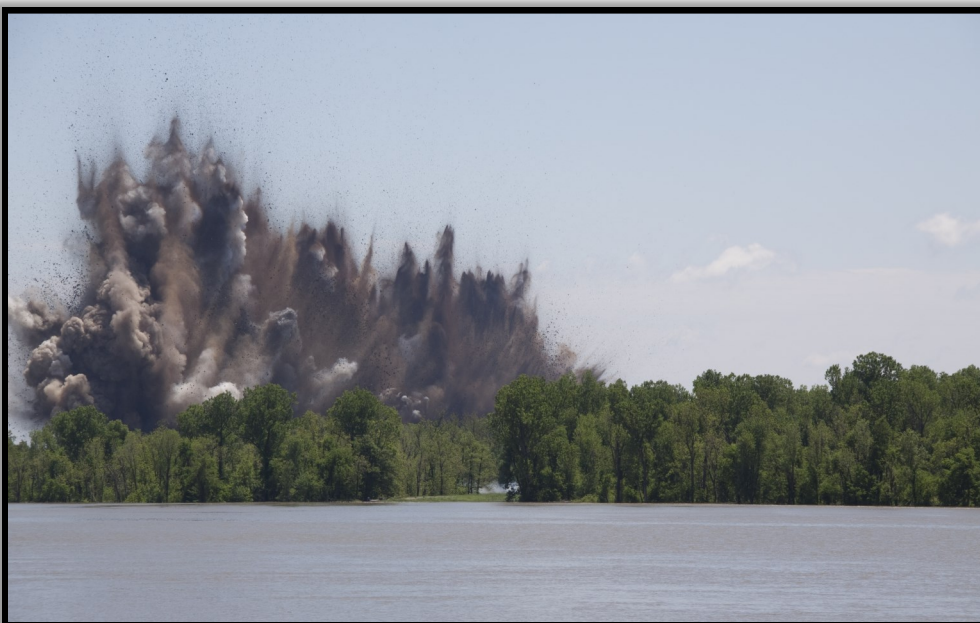
2011 flood - blast for middle crevasse at Birds Point-New Madrid floodway
