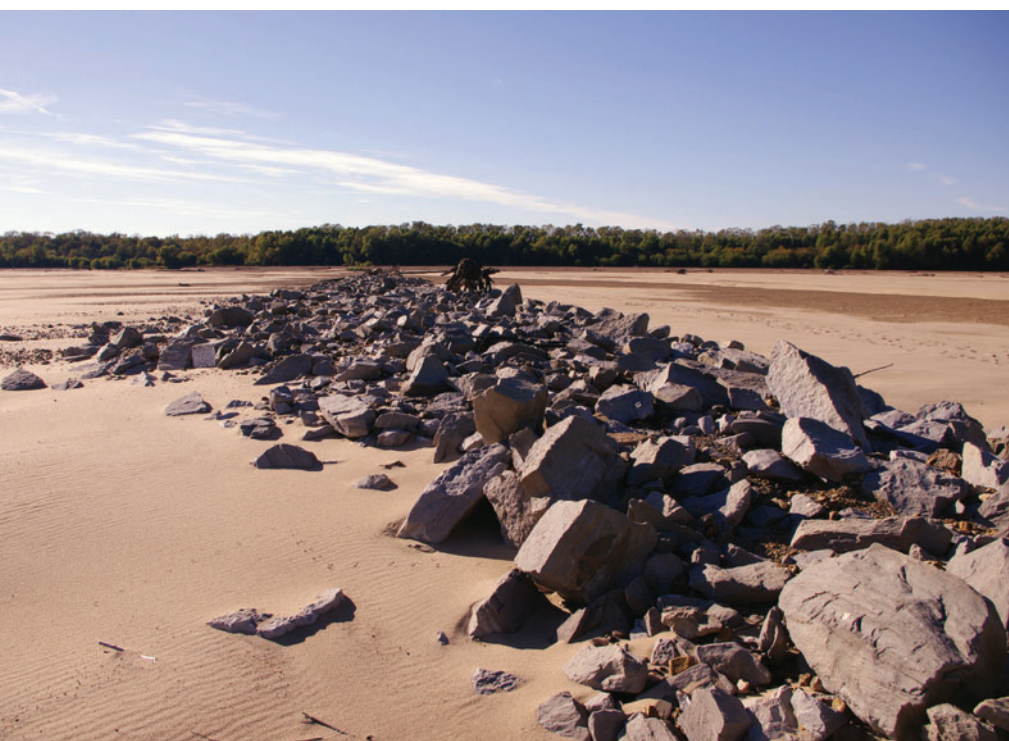
A stone dike structure prior to the 2013 construction. It was constructed in the 1970's within the Vicksburg District in Bolivar County and has silted in over time.
