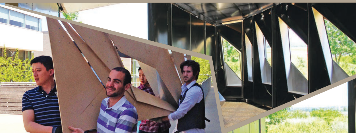
LEFT: Students carry the final full-scale prototype of one exterior panel to their final review in May 2013. MIDDLE: The nearly complete interior just before the opening in August 2013. RIGHT: Students testing the final prototype in May 2013. They tested both the functionality of the diagonal apertures, here testing visibility with a birding scope, and ensured proper fit and installation sequence.
