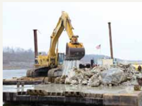
LEFT: Contractors load a spud barge near Thebes, Ill., during efforts to blast 890 cubic yards of limestone from the Mississippi River navigation channel. ABOVE: Geologists say that in ancient times, the pinnacles were part of a massive waterfall that fell at twice the height of Niagara Falls from the river into the Gulf of Mexico.
