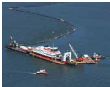
FROM TOP: Birds flock above new islands and other land created by dredged sediment. A dredge works to create land in a wildlife refuge.
