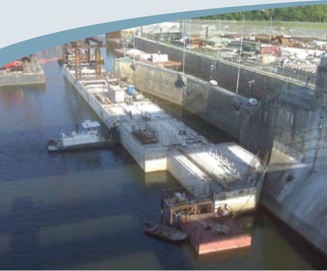
Construction underway at the Chickamauga lock in the Nashville District of the U.S. Army Corps of Engineers. Portions of the new lock are being made from prefabricated concrete boxes using in-the-wet construction methods.
