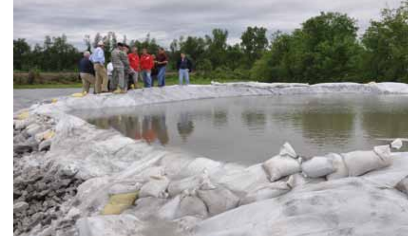
A crew monitors a massive, pond-sized sand boil in Cairo, Ill., in the midst of the Great Flood of 2011.
