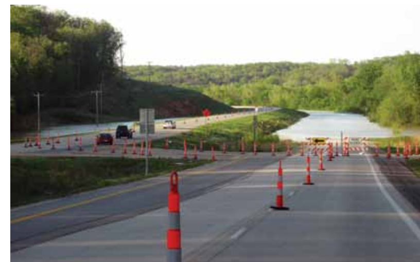
ABOVE: Newly raised Highway 67, flood-proofed through ARRA funds.
