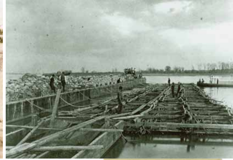
ABOVE, FROM LEFT: Early levee construction, around 1910. Workers construct a willow mat that will be loaded with rock for channel protection or wing dike formation.
