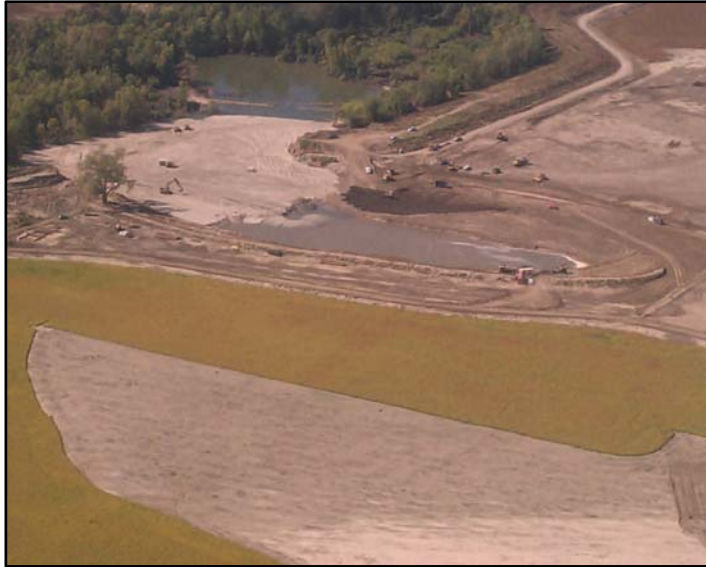
Photograph 7. Repair Activity at Middle Crevasse of BPNM Floodway his is one of many locations with aggressive repair construction activity
