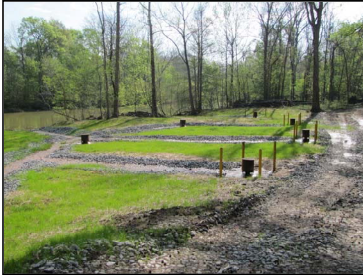
Photograph 8. Buck Chute Mainline Levee Seepage Repair located just north of Vicksburg, MS
