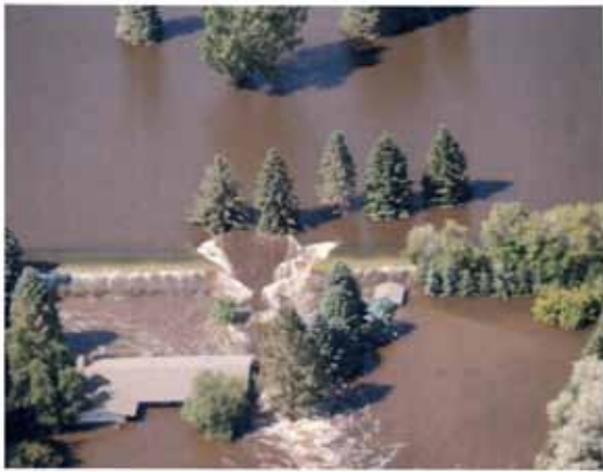
Figure (4) Levee breach on Souris River at Minot, ND
