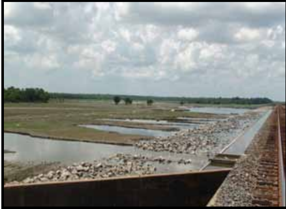
Figure (10) Scour at Morganza Floodway
