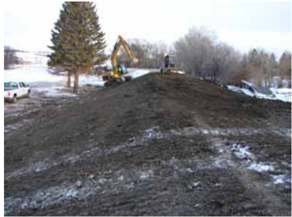
Figure (5) Levee construction at Minot, ND
