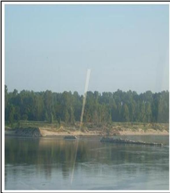
Photograph V-1. Typical Damage to a Dike
