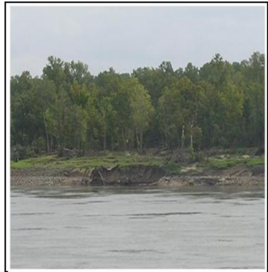
Photograph V-2. Typical Damage to Revetment
