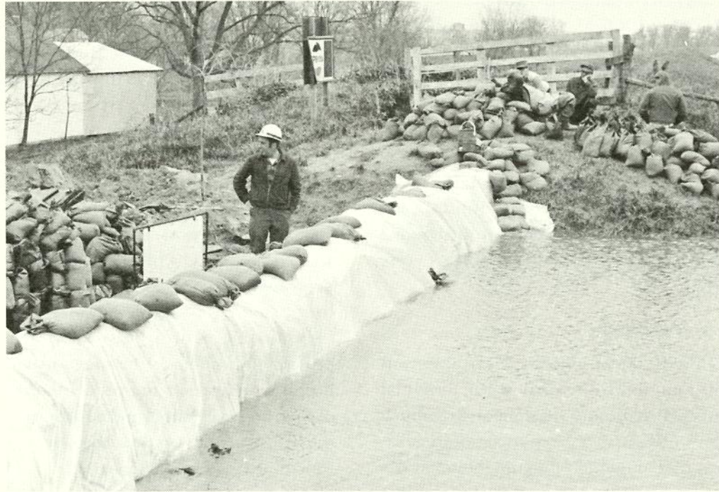
Kampsville Ferry Landing closure, Highway 108 and Eldred levee, 26 April 1973
