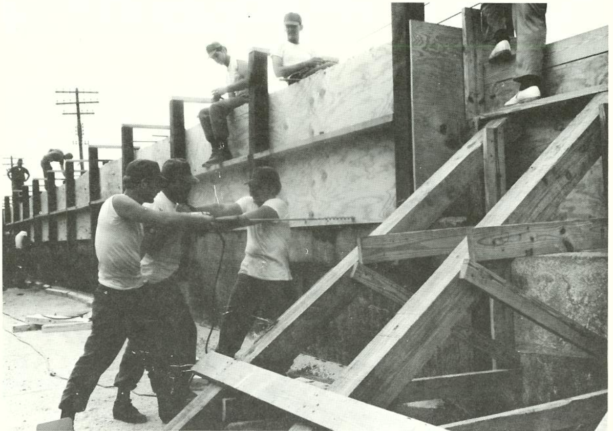
Construction of mudboxes atop floodwall at Morgan City, Louisiana, by U. S. 5th Army, 62d Engineer Battalion, Fort Hood, Texas
