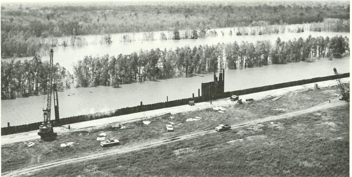
Steel sheet piling used north of Morgan City, Louisiana, East Atchafalaya Basin protection levee
