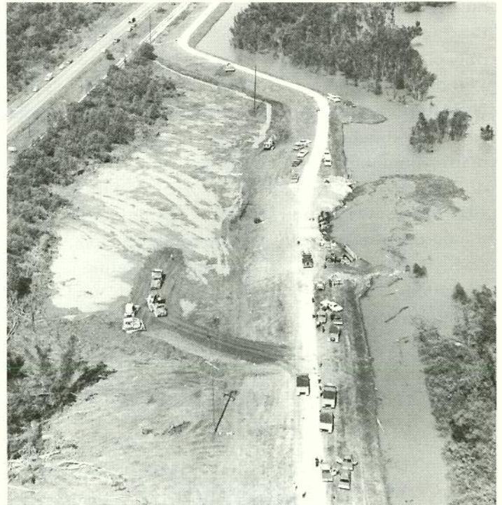
Bank failure and construction of levee setback, mile 35 AHP, Mississippi River levee, vicinity of Nairn, Louisiana
