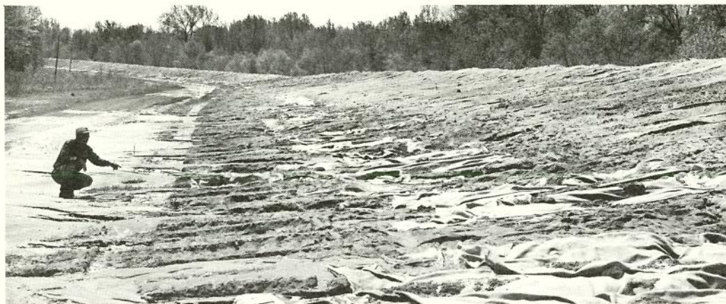
Sny Island drainage district, burlap used to stop erosion caused by seepage on land side of levee upstream from pump station No. 1, looking downstream, 28 April 1973
