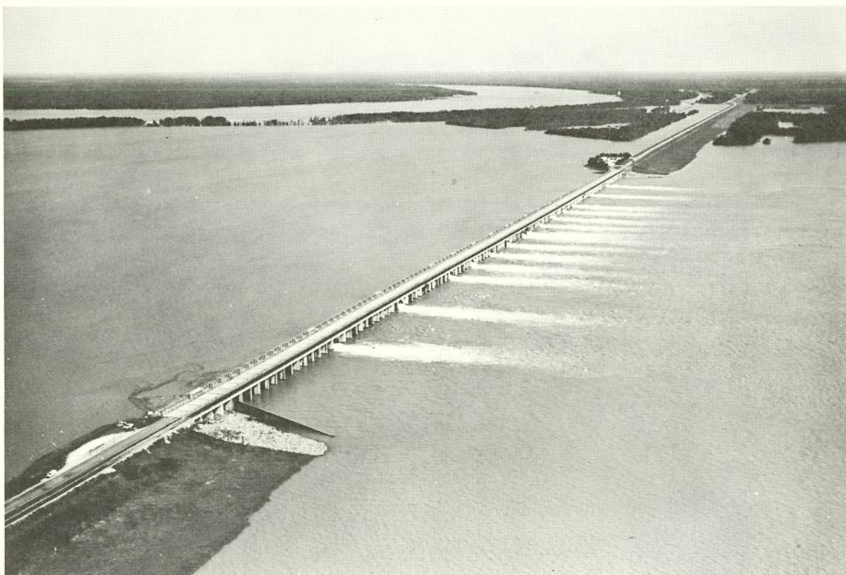
Morganza Control Structure during operation
