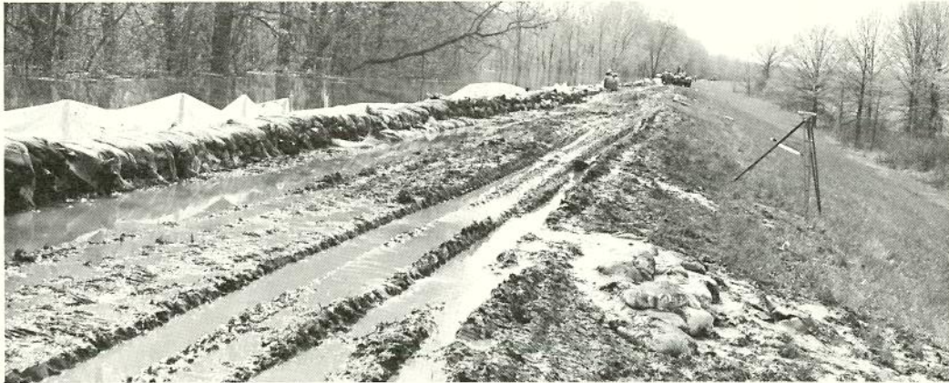
Fabius drainage district, north of pumping station on Fabius levee, looking upstream, 23 April 1973
