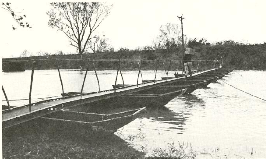
Emergency pontoon foot bridge assembled by Army personnel from Fort Leonard Wood, Missouri
