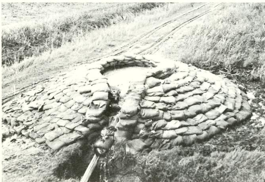
Typical example of a sand boil, ringed with sandbags to create enough head to slow the flow
