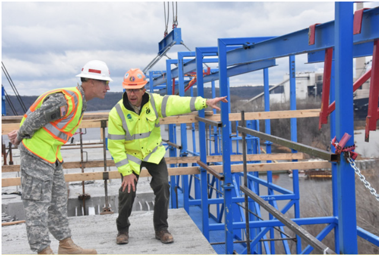
(Left) Maj. Gen. Michael Wehr, MVD commander, tours the construction site of the St. Croix River Bridge, which will connect Oak Park Heights, Minnesota, and St. Joseph, Wisconsin, when it is completed in the fall of 2016. (USACE photo by Ben Watson)
