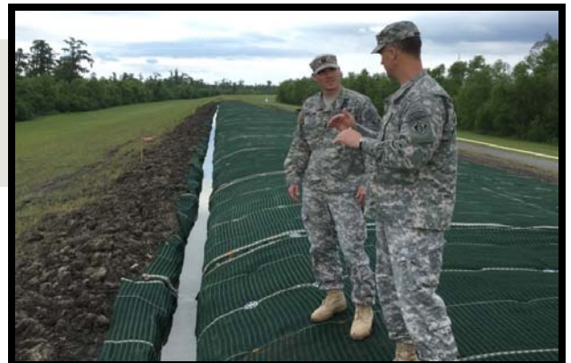
Capt. Matt Miller briefing Maj. Gen. Mike Wehr on armoring installation in the vicinity of Bonnet Carre' Spillway.
