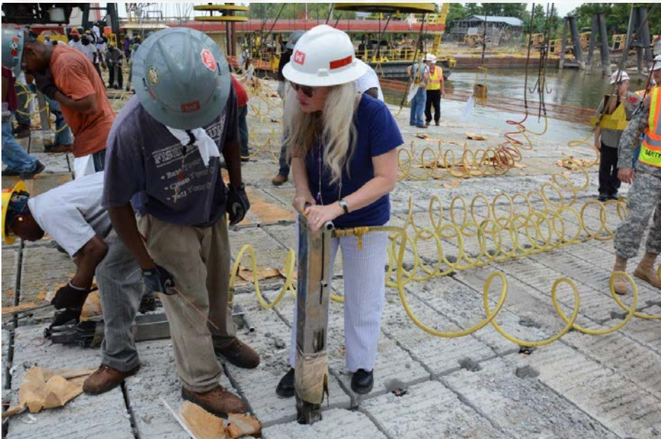
During a visit on the Mat Sinking Unit in Vicksburg, Miss., the Honorable Norma Jean Mattei, Ph.D., civilian Mississippi River Commission member/civil engineer, helps one of the crew members tie together blocks of concrete that make up the revetment mattress on the MSU during the MRC's low-water inspection trip.
