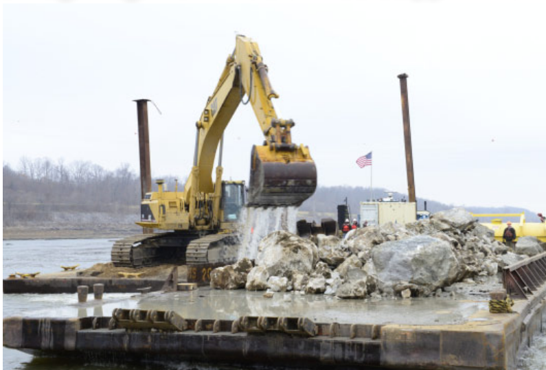
Loading a spud barge —The removal of 890 cubic yards of limestone from the navigation channel on the Mississippi River near Thebes, Ill., began Dec. 17, 2012. This is just one phase of the action the Corps is taking to improve the navigation channel for the river industry.
