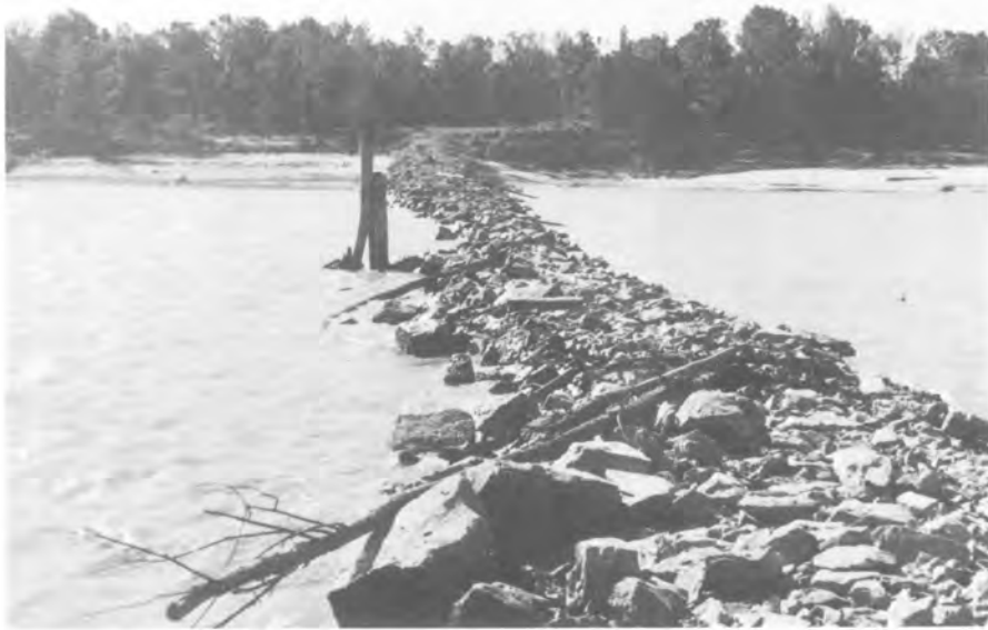
Photo 3. Togo Island Dike No. 2, mile 416, 23 September 1975
