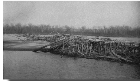
Early dike works
