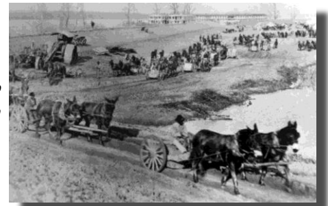
Early levee construction
